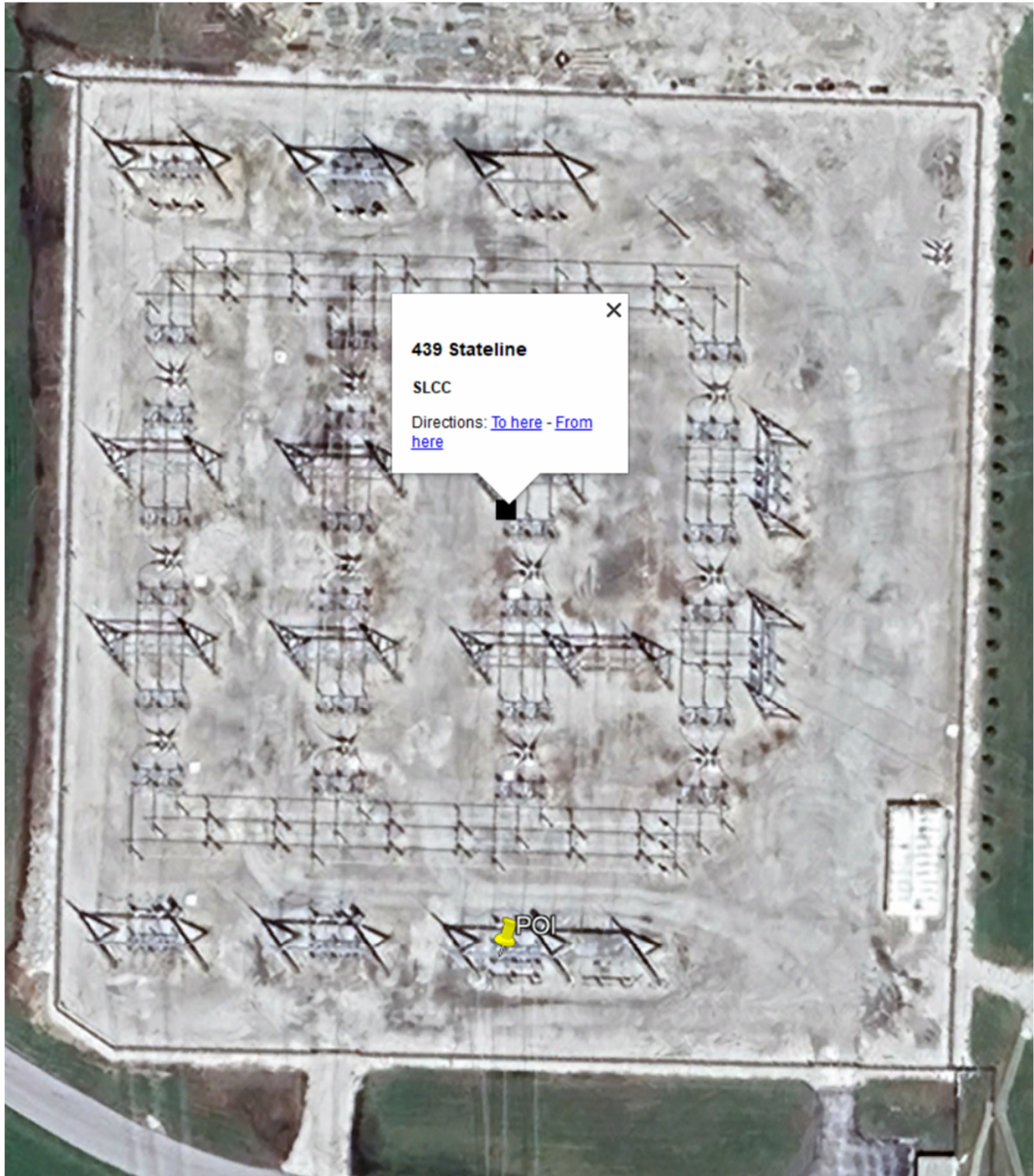
Figure 1 – State Line Substation and POI location
